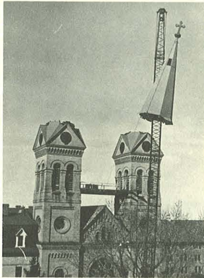
Removing twin towers of old church
