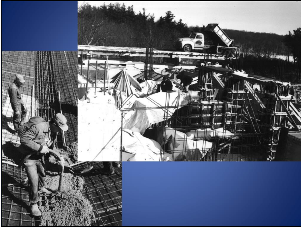
Lots of rebar, lots of cement.
