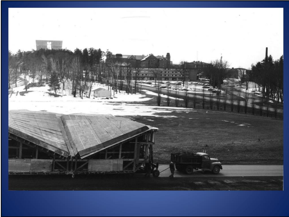
Transporting the form used to cast the 20 dorm roof modules?
