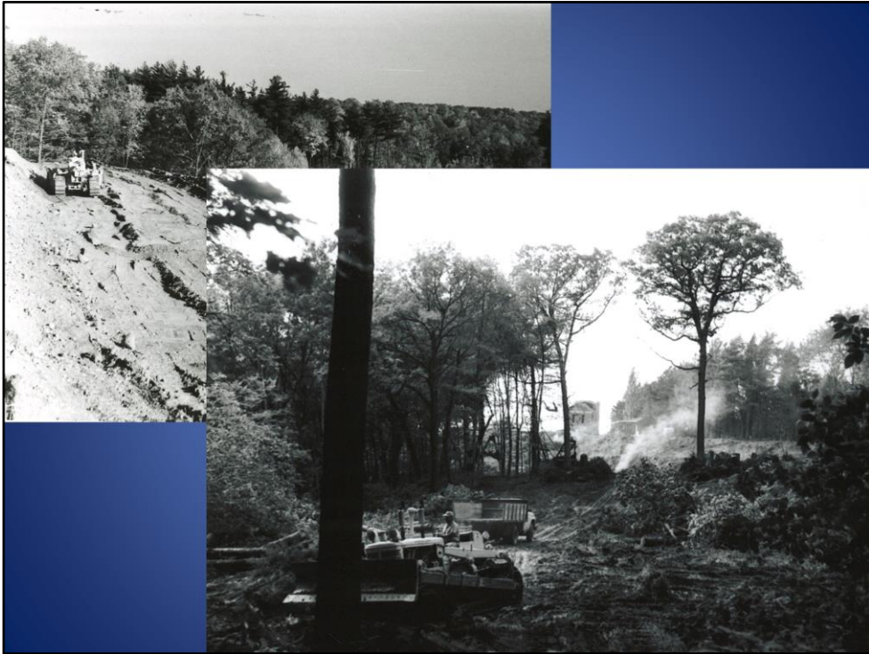
The site is logged and cleared.
