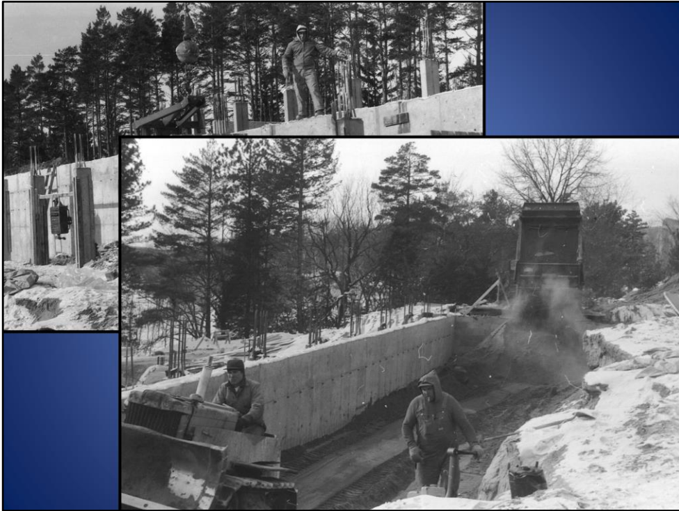
Cement work continues through the winter cold.
